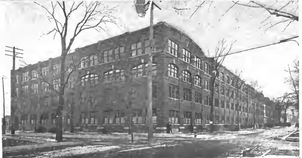
Two more examples of the type of buildings erected and occupied by the automobile manufacturing companies of Detroit. The illustrations furnish a very good idea of the magnitude of the plants, which turn out more automobiles than all the factories of Europe combined
